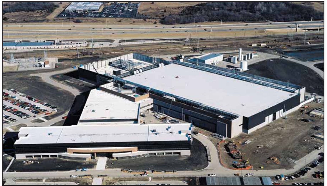
RFAB photo shows administration building, facing Renner Road (in foreground), linked to the manufacturing facility.
